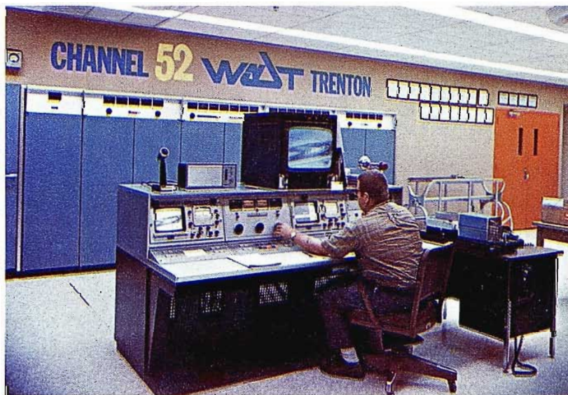
A TTU-60, 60 kW UHF transmitter is installed at each of the four statewide NJPB transmitting locations. The WNJT-TV, Ch. 52, Trenton facility illustrated is typical.
