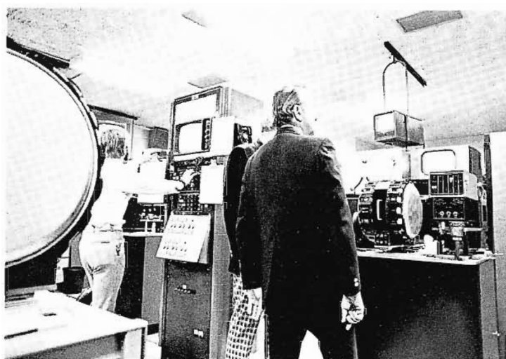
In the Film Room, machine controls for the four TK-27 film systems are remoted to a central panel. A second set of remote panels is in Master Control.
