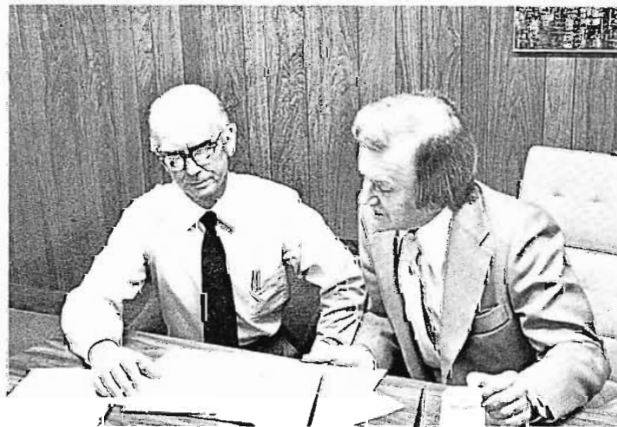
Chief Engineer E. Dennis White, left, discusses station plans with General Manager Donald Moeller.
