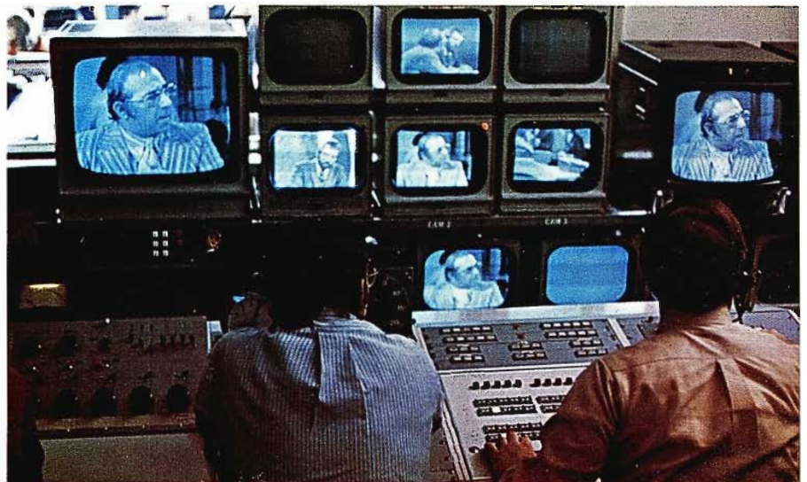
Production console for one of two fully equipped studios at Jerseyvision's teleproduction center in Trenton.
