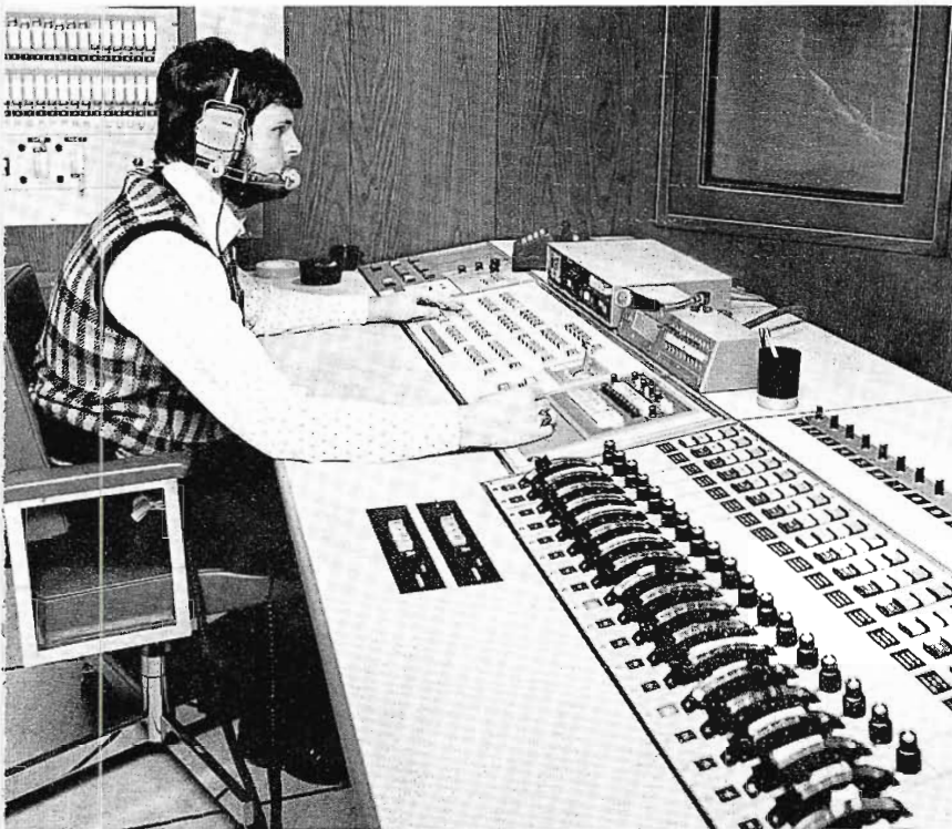
Director, left, calls on special effects of TS-51 System 14 Video Switcher. Four bus unit has two bus panels assigned to mix and effects and two for preset/preview and program. Engineer, right, operates joystick control for #2 studio camera while also keeping a hand on the audio fader controls. The BC-100, with 18 mike inputs and 2 channels out, is an audio-follow-video system that works especially well in quick-turnaround news shows and in cuts between local and remotes on network productions.
